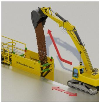
Continue to backfill and compact in stages.
