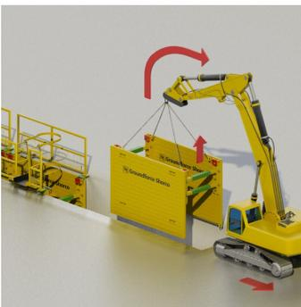
Attach a four leg chain to the lifting points and lift clear of the excavation.
