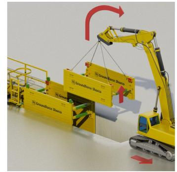
Attach a four leg lifting chain to the lifting points and lift the top box and set carefully to one side.
