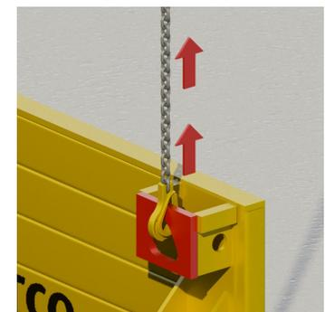
Re-attach the single leg chain and continue to shuffle the box out of the trench in 150mm stages.
