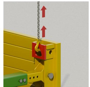
7. Using a single heavy duty chain, attach to each corner of the box and lift by no more than 150mm each time. **Do not snatch the chain**
