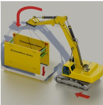
Lower the assembled box into the guide trench.
