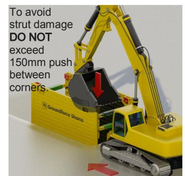
To avoid strut damage **DO NOT** exceed 150mm push between corners.
