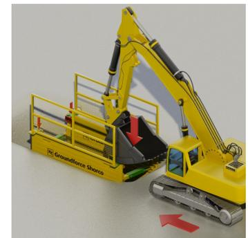
Excavate to the required depth. Push separately on the green bracket at each corner, avoiding damage to the handrail system.
