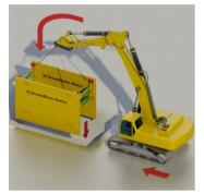
Lower the assembled box into the guide trench.
