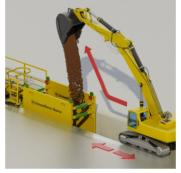
Continue to backfill and compact in stages.
