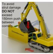
Push down on each corner of the box using the excavator bucket.
