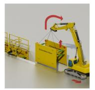
Attach a four leg chain to the lifting points and lift clear of the excavation.
