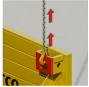
Re-attach the single leg chain and continue to shuffle the box out of the trench in 150mm stages.
